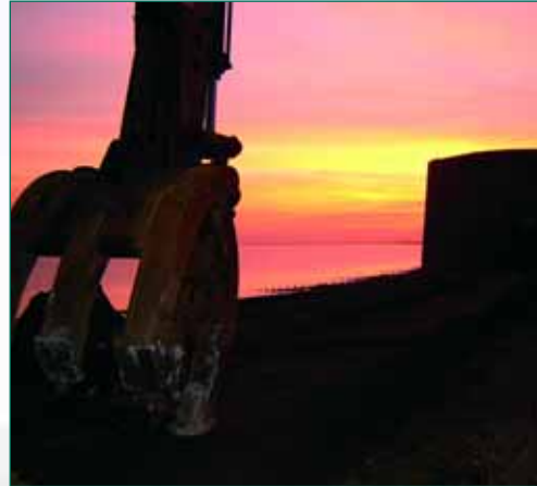
Sea defence repairs at DTE South East.
