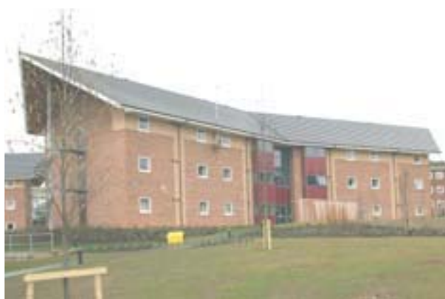
Completed SLAM accommodation at St. David's Barracks
