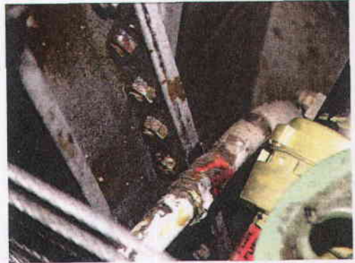
Figure D-4; A(Inv), Chafing, Zone 514, APU fuel feed chafing on bulkhead and fairlead nut
