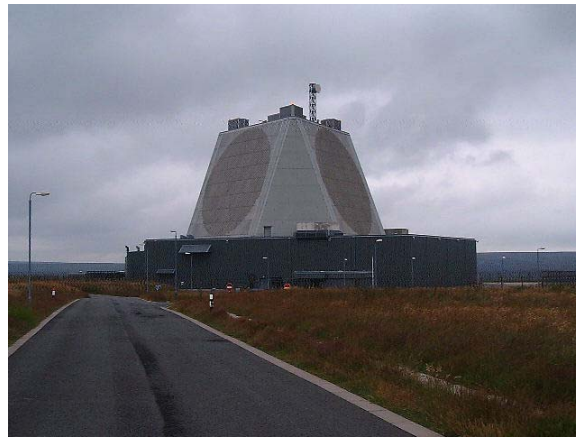
View of EWR from south
