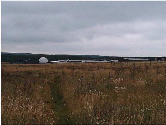
Satellite Communications Radome
